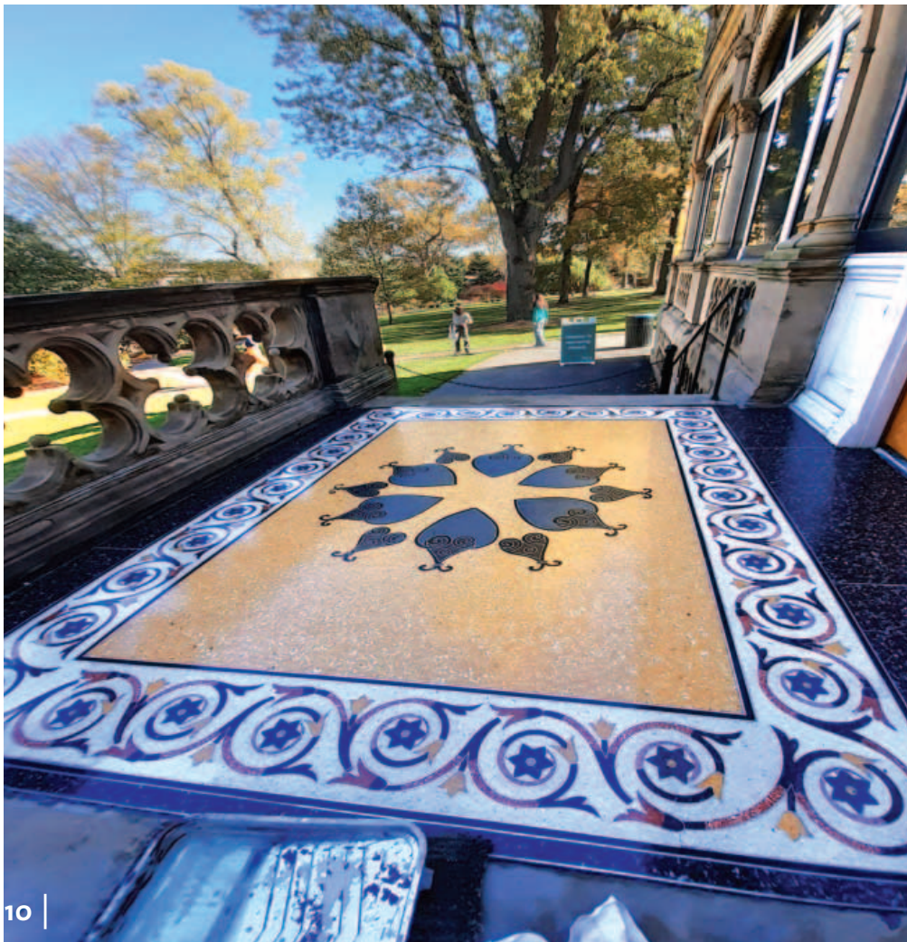
Left: Terrazzo restoration completed at the entrance of Clayton. Background: Detail of conserved terrazzo fragments prior to reinstallation.
