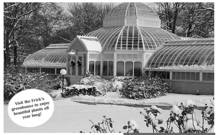
Greenhouses work because the sun's rays come through the glass roof as light energy. When it hits the plants and soil of the greenhouse, the light energy changes into heat energy. Heat energy can't get back out through the glass as easily as light energy came in, so the temperature stays higher inside.
